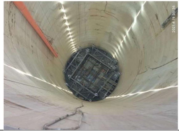
Installation of the shelter interior modules
